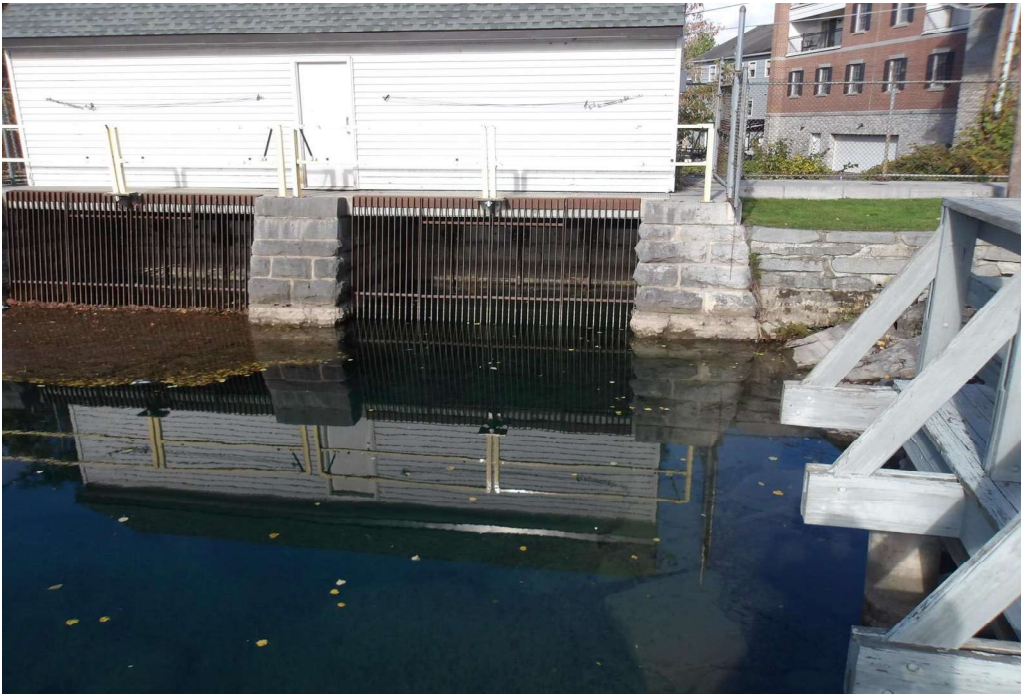
Photo 10 Dam ID# 073-0355 Skaneateles Lake Dam 10/23/2023 Right upstream face of the dam.
