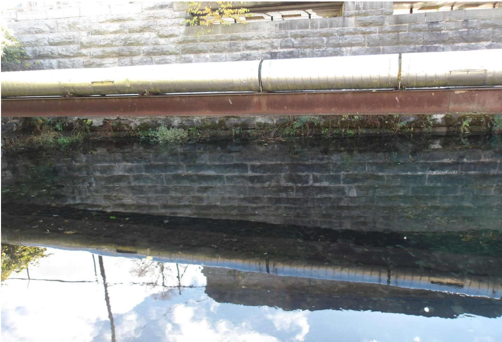
Photo 4 Dam ID# 073-0355 Skaneateles Lake Dam 10/23/2023 Right Downstream groin.
