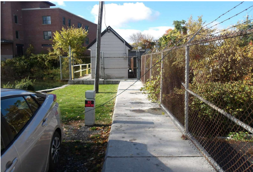
Photo 2 Dam ID# 073-0355 Skaneateles Lake Dam 10/23/2023 Dam crest looking left.
