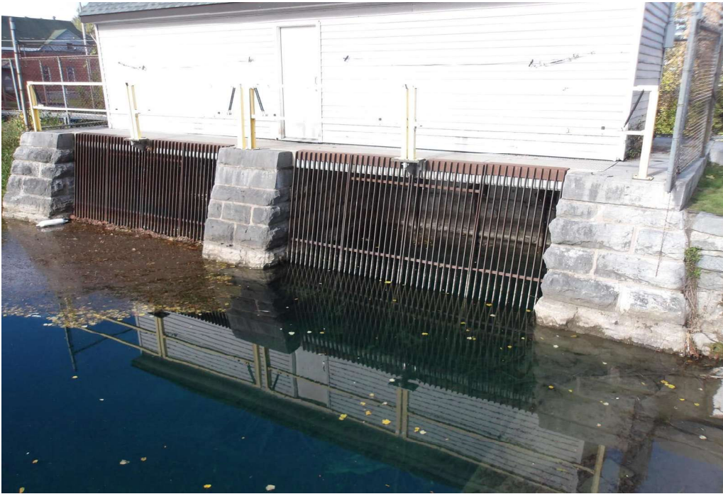
Photo 1 Dam ID# 073-0355 Skaneateles Lake Dam 10/23/2023 Upstream face of the dam.
