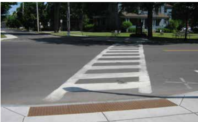
The crosswalk at the West Lake Street / Hannum Street intersection across U.S. 20 is uncontrolled.
