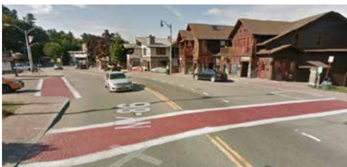
Brick pavers are frequently used to make crosswalks visually distinct from the surrounding pavement. They are used at many crosswalks in Auburn (top photo) and Lake Placid (bottom photo). (Photo: Google Streetview)
