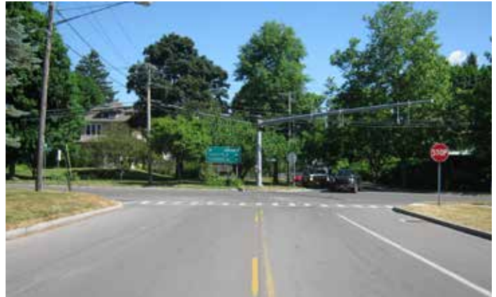
The northbound Kane Avenue approach is controlled by a stop sign and a yellow/red flashing signal.
