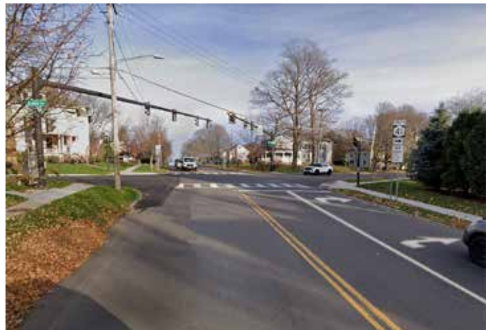
This photosimulation shows eastbound U.S. 20 with a proposed dedicated right-turn lane to southbound East Lake Road.
