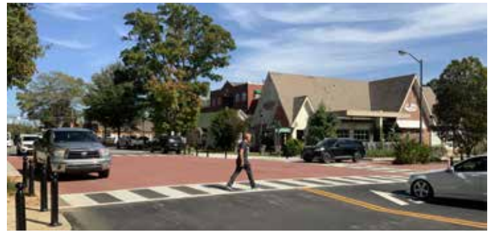
Raised intersection in Matthews, North Carolina. (Photo Alta Planning + Design)
