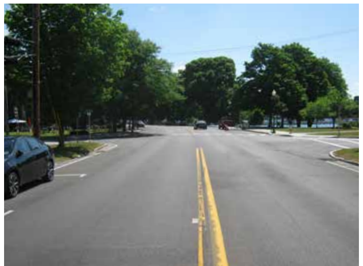
U.S. 20 eastbound approach at the West Lake Street intersection.
