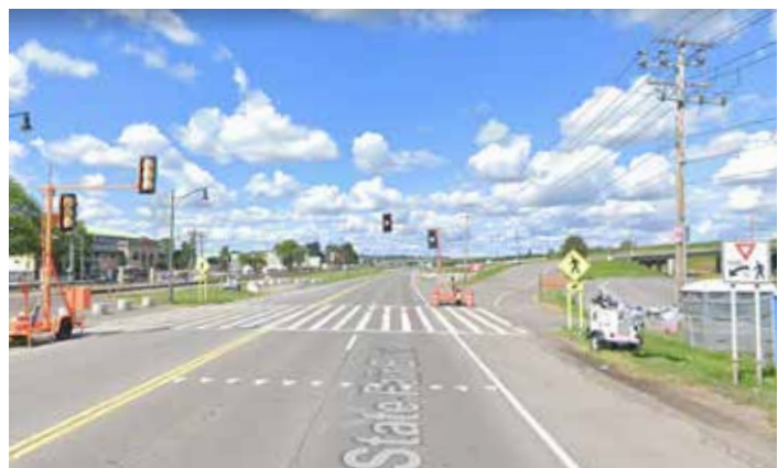
Temporary 3-color signal at crosswalk on State Fair Boulevard. (Photo: Google)
