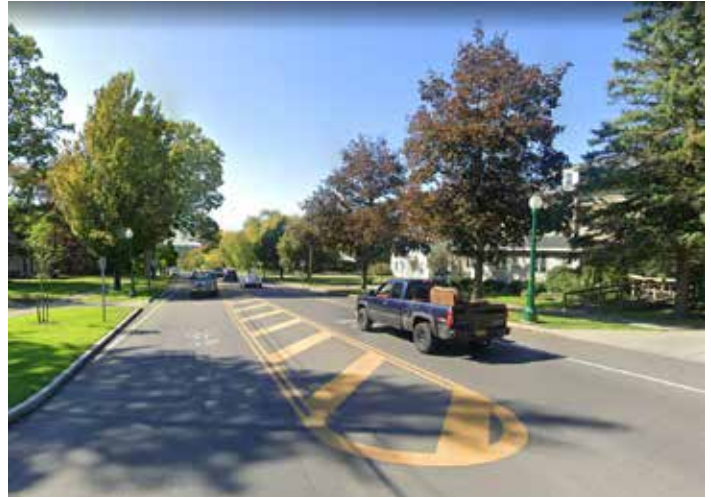
Example of a painted median (Auburn, NY). (Photo: Google Streetview)
