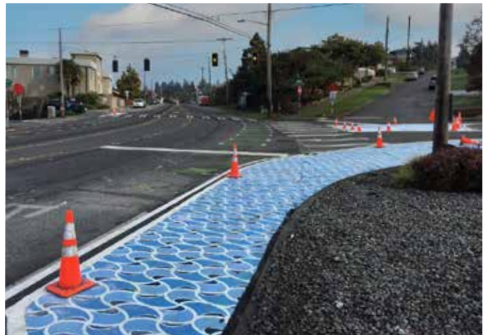
Painted curb extensions can be aesthetically pleasing while providing a benefit to pedestrians. (Photo: Seattle Department of Transportation)
