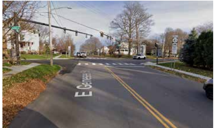
Existing conditions on U.S. 20 eastbound at the East Lake Street (Route 41) intersection.
