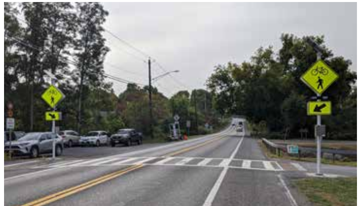
A set of rectangular rapid flashing beacons (RRFB) across Warners Road in Camillus, along the Empire State Trail.
