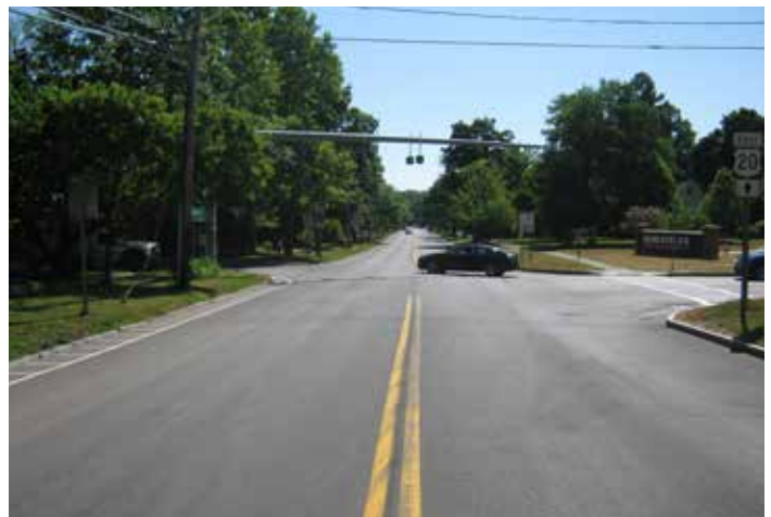
Flashing yellow lights on the eastbound approach of U.S.20 at the Kane/Orchard intersection.
