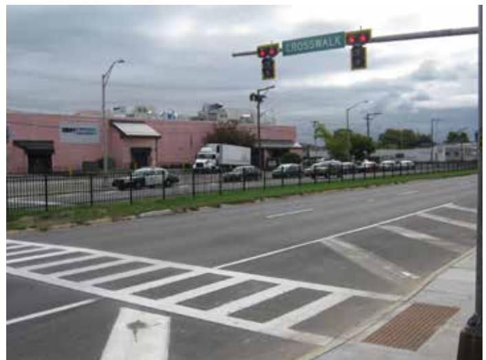
A pedestrian hybrid beacon (PHB) on West Street in the City of Syracuse.
