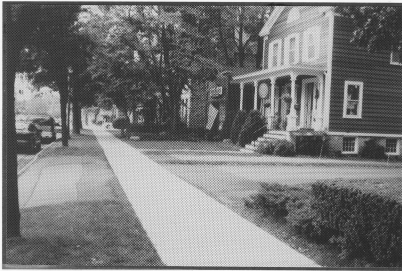
Encouraged: Sidewalks should continue across driveway cuts.
