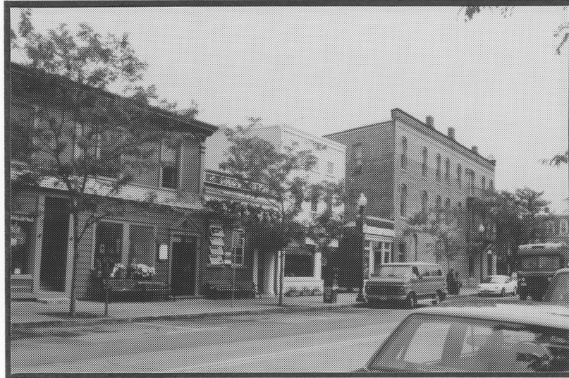
Single-story buildings break the continuity of the street wall.
